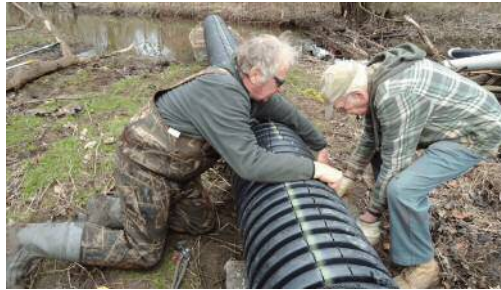
Connecting the pipes
