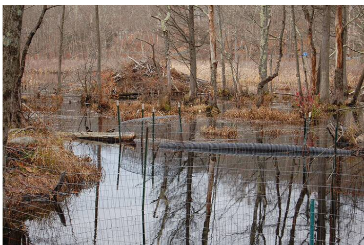
On this property owned by the Cumberland Land Trust, the organization installed plastic pipes and fencing to address the flooding problems beavers created. There is large beaver lodge in the background. (Todd McLeish/ecoRI News)
