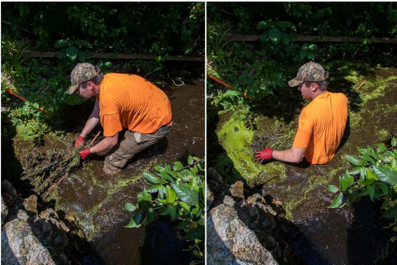
Left: Water flow through the culvert on the other side of the marsh is only knee high. Right: Water is finally free to flow through the culvert after John Egan removes the last bits of debris left by beavers. (Jesse Costa/WBUR)
