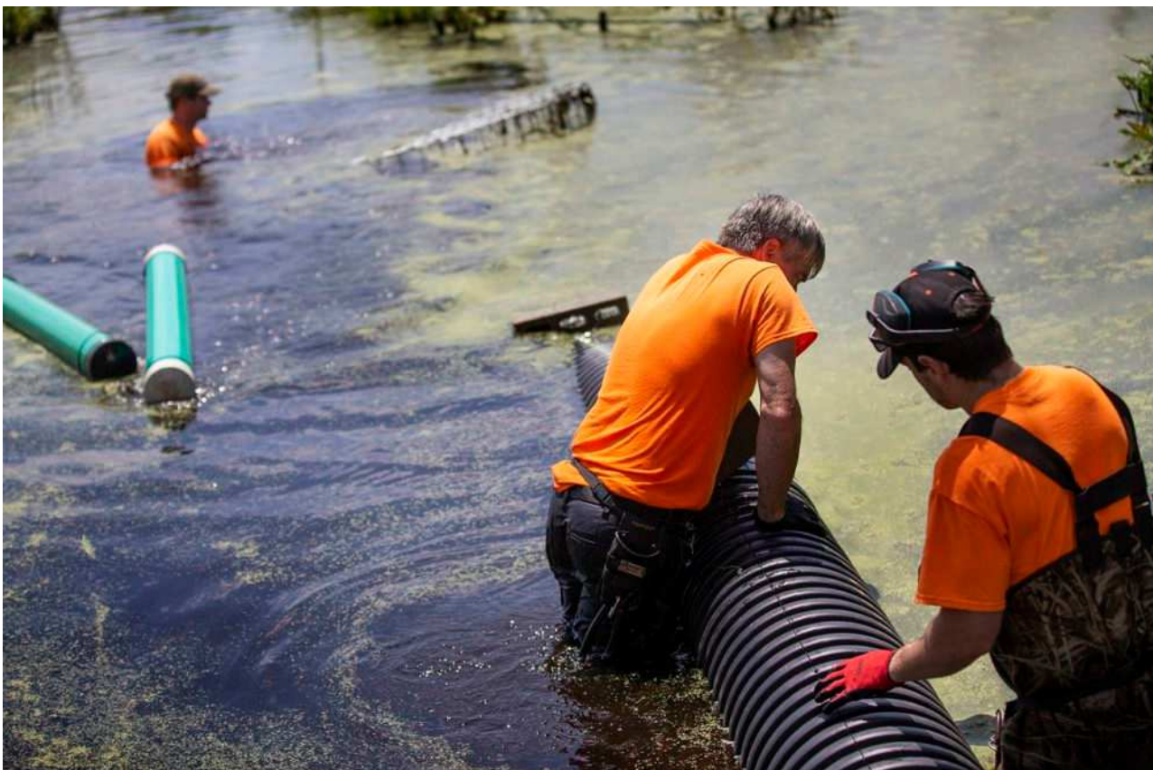
Mike Callahan and Edward Beattie submerge the pipe as John Egan sinks the cage to the
