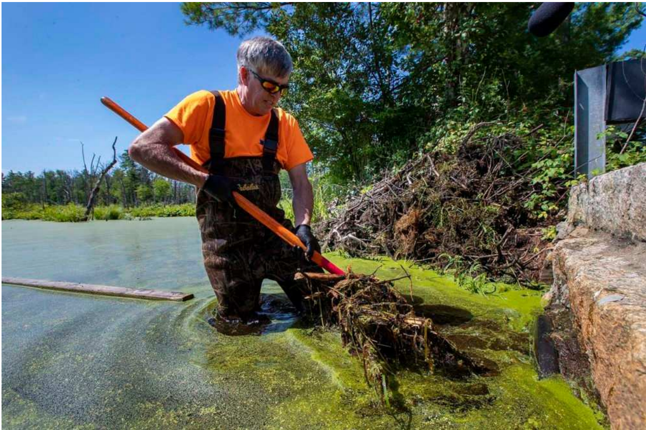
Mike Callahan, owner of Beaver Solutions, pulls out debris from a culvert beavers dammed up on Causeway Street in Millis. (Jesse Costa/WBUR)
