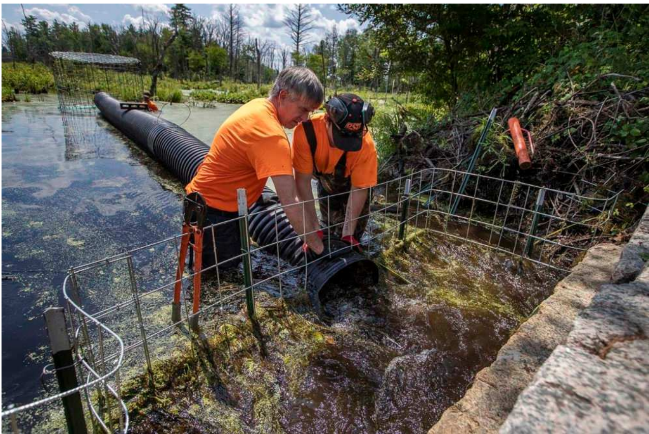
Mike Callahan and John Egan place the pipe into position during the installation of the flow device on Causeway Street. (Jesse Costa/WBUR)
